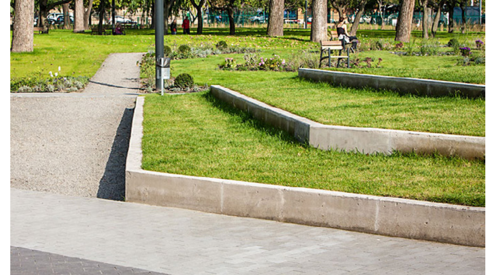
Insitu concrete terracing
